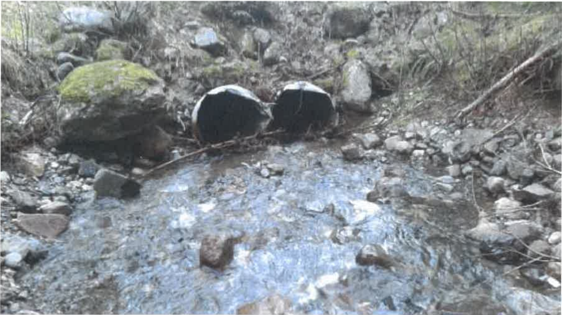
Above: Two 36" metal culverts where creek leaves the site on the east and passes under the Silver Fir parking lot to the east Below: Tunnel Creek upstream of two 36" culverts on east side of site.
